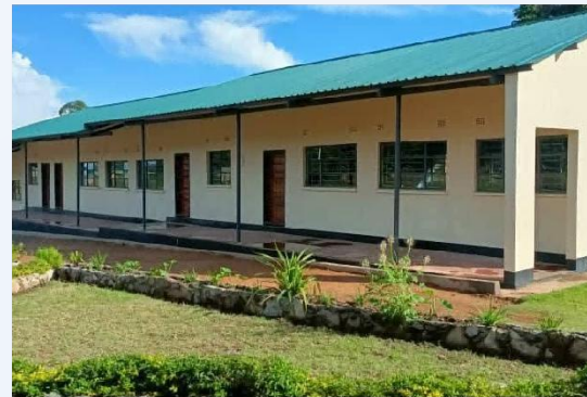
Zambia: Lubambe Company Constructs Classrooms for Local Schools
