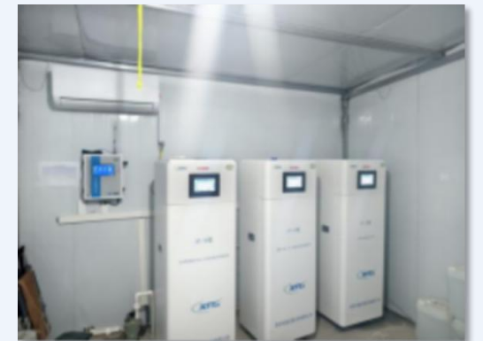
Installation of flow meters at the inlet and outlet, and online monitoring systems at the mine water treatment station
